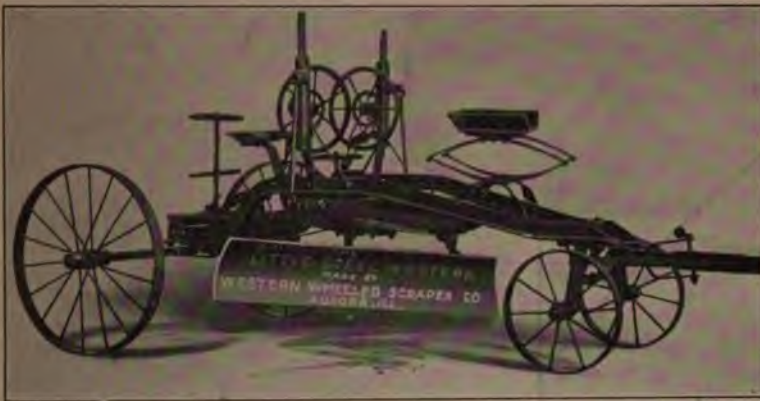
Light Four-wheel Grader. Figure 11.
